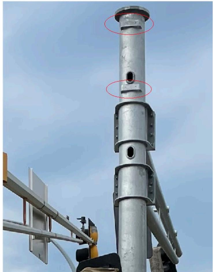
Figure 3-5 Mounting Straps on the TS Pole for Mounting the CCTV Cabinet
