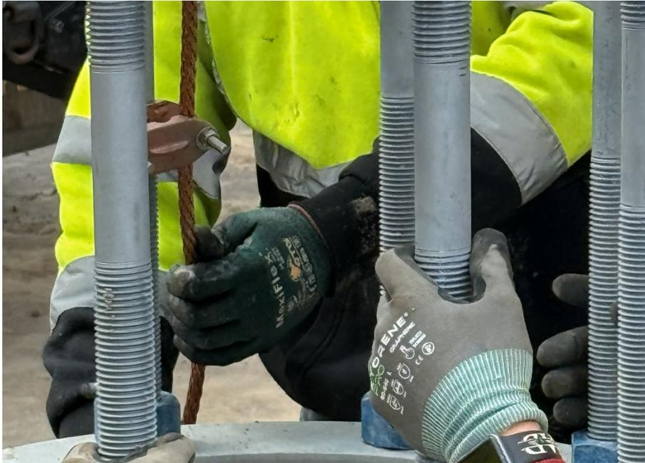
Figure 2-24 Dead End LP Conductor After Connecting With U-Bolt Bonding Clamp
