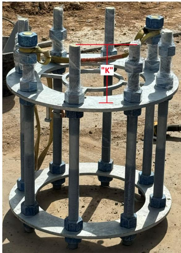
The nuts used to hold down the upper anchor rod template are the leveling nuts for the pole. Make sure not to use the F436 structural flat washers that are part of the anchor rod hardware between the hex nuts and the upper and lower anchor rod templates. The washers are specifically for the pole anchor rod connections.
