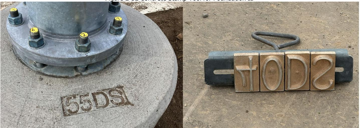
Stamp the concrete in two separate areas outside of the anchor rod circle that will not be covered by the pole base plate. Ensure imprinted ID in the concrete is legible.
