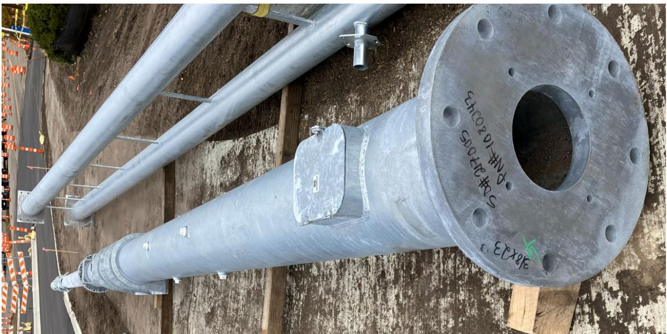
Those who are familiar with installing PA series poles may have at some point raked the poles on the foundations by raising the leveling nuts up on the side of the mast arm. Raking the pole helps with deflection especially when the longer mast arms 45' to 55' are installed. The loading of the arms can cause the structure to
