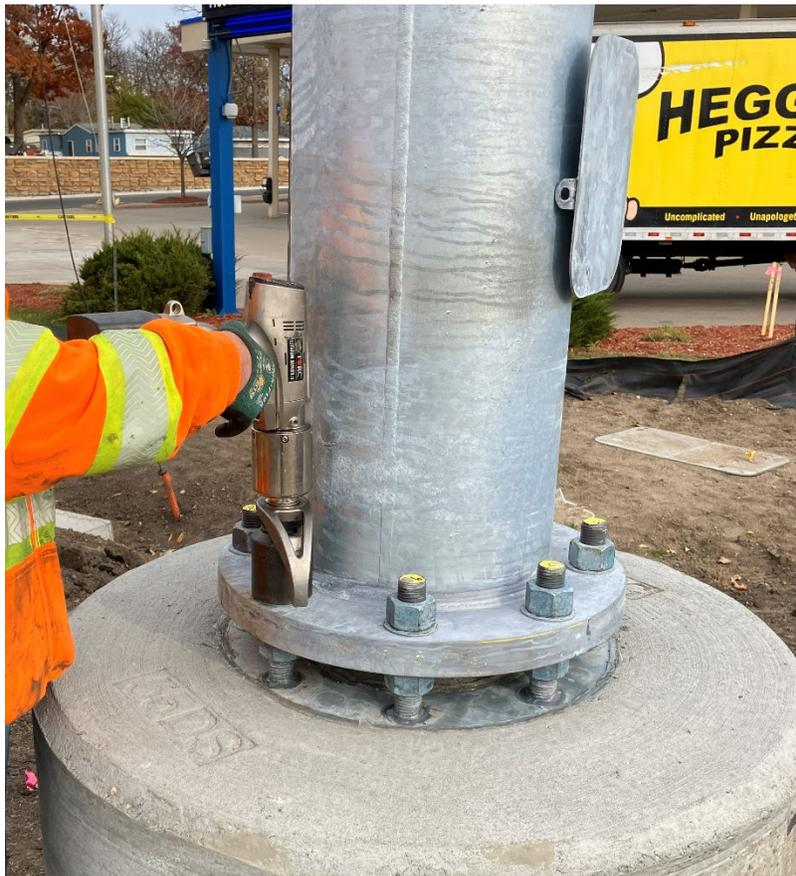
The cordless battery torque wrenches have a “rundown” feature, or snug setting. Because of this, the 20% torque value cycle for typically tightening anchor rods and bolts has been eliminated for tightening TS pole anchor rods and bolts and replaced with this rundown or snug wrench setting. One of torque wrenches the
